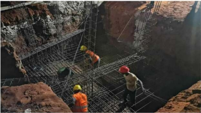
NIGHT FOUNDATION WORKS
